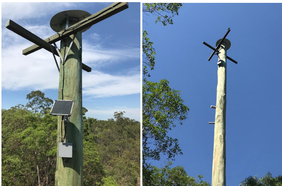
Photo Plate 1: Example of horizontal crossbars installed at the top of glide poles. Depending on launch direction, 1 or 2 crossbars may be required. PVC pipe refuge observed in the 2 nd photo. Photo credit: A. Marks.
